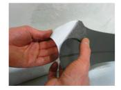
L-foam 18 is placed in square, at the junction between the horizontally unrolled underlay and the wall.
